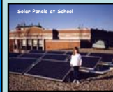
Solar Panels at School
